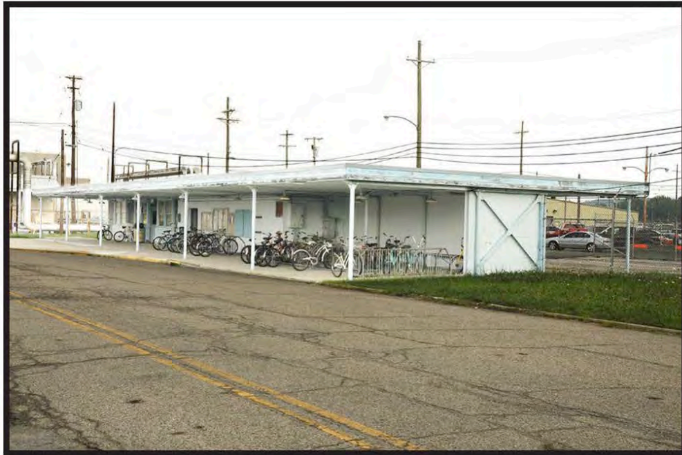
Figure 3: South Side of the X-108B Security Portal, August 5, 2011, Facing Northeast
