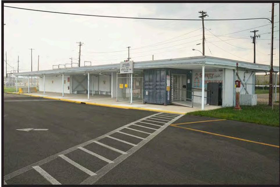
Figure 2: North Side of the X-108B Security Portal, August 5, 2011, Facing Southwest
