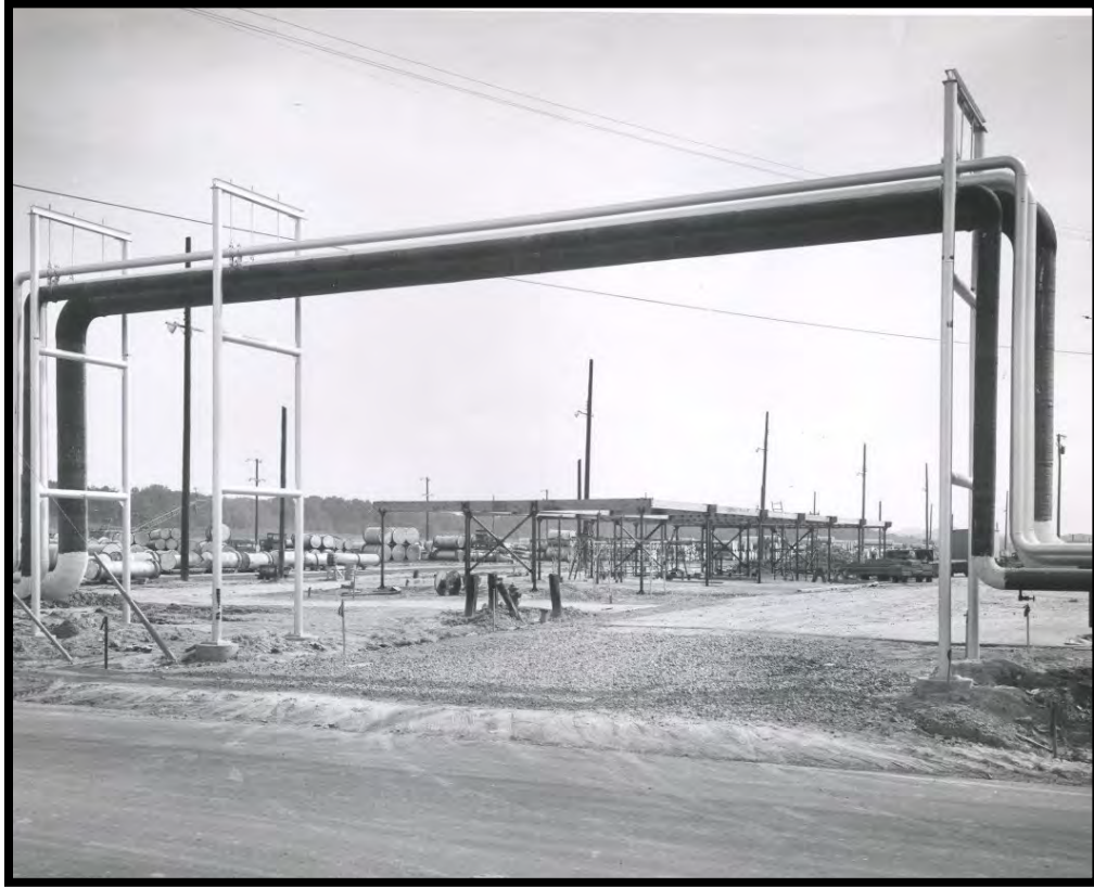
Figure 4: Looking Northeast at X-108B Security Portal Construction, 1955
