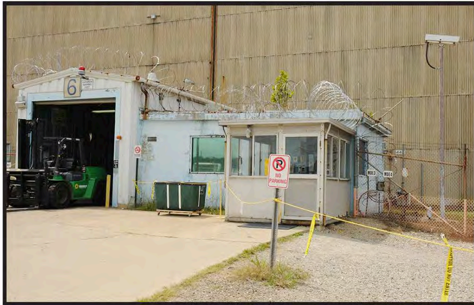
Figure 2: North Side of the X-111A Special Nuclear Materials Monitoring Portal, August 2014, Facing Southwest
