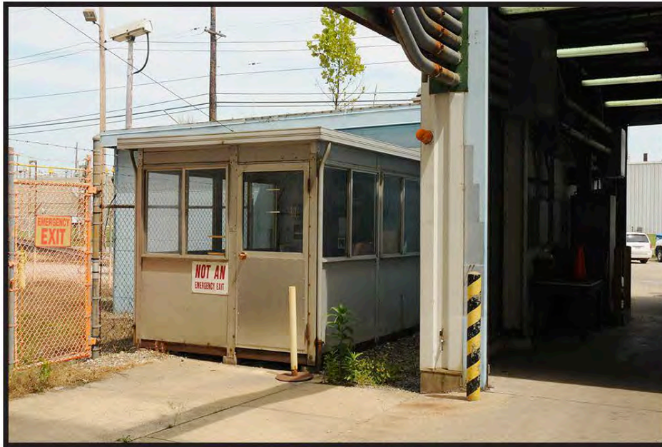
Figure 3: South Side of the X-111A Special Nuclear Materials Monitoring Portal, August 2014, Facing Northeast
