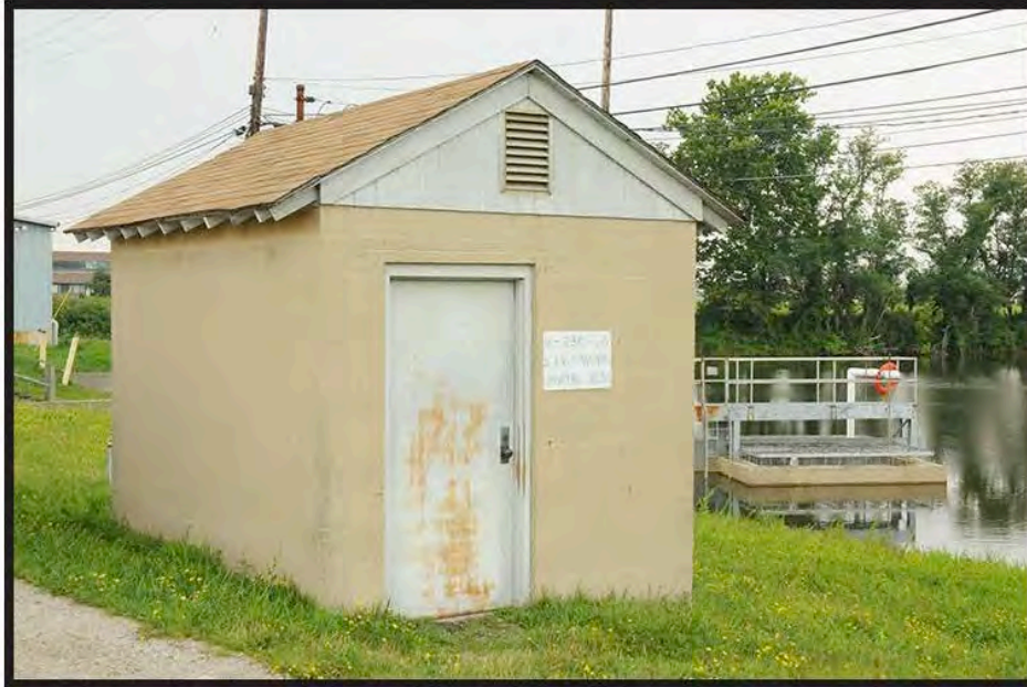
Figure 2: South Side of the X-230J2 South Environmental Sample Station, August 2014, Facing Northwest
