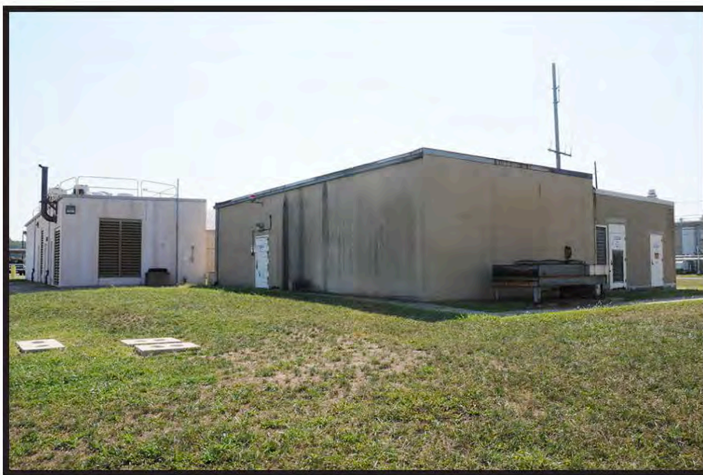
Figure 2: North Side of the X-300A Process Monitoring Building, August 2014, Facing Southeast
