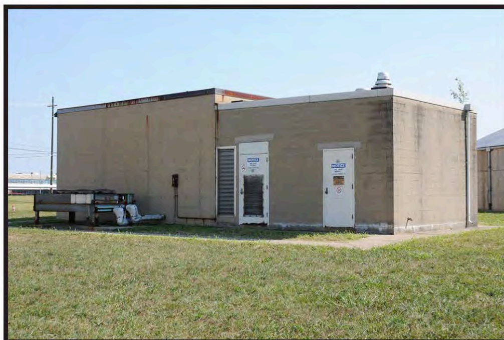
Figure 3: South Side of the X-300A Process Monitoring Building, August 2014, Facing Northeast
