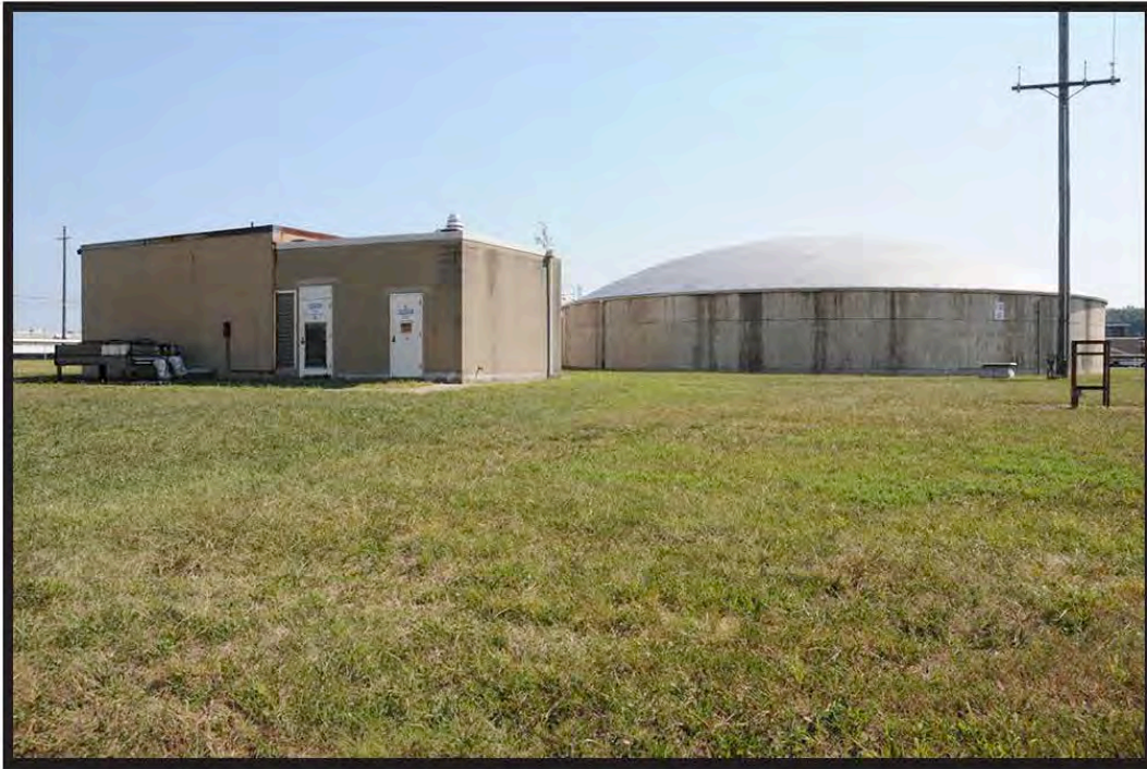
Figure 4: South Side of the X-300A Process Monitoring Building, August 2014, Facing Northeast
