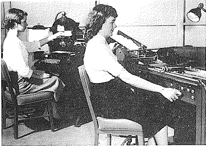
PANSY CARTER, left, is making a new address plate on the Graph-O-Type. Lillian Cutlip runs the plates through the address-o-graph after they have been made by the graph-o-type machine. The address-o-graph machine has an automatic feed and can address communications at the rate of 100 pieces a minute, thus speeding up the process of mailing. The two new machines, located in the mail department, went into operation last month.
