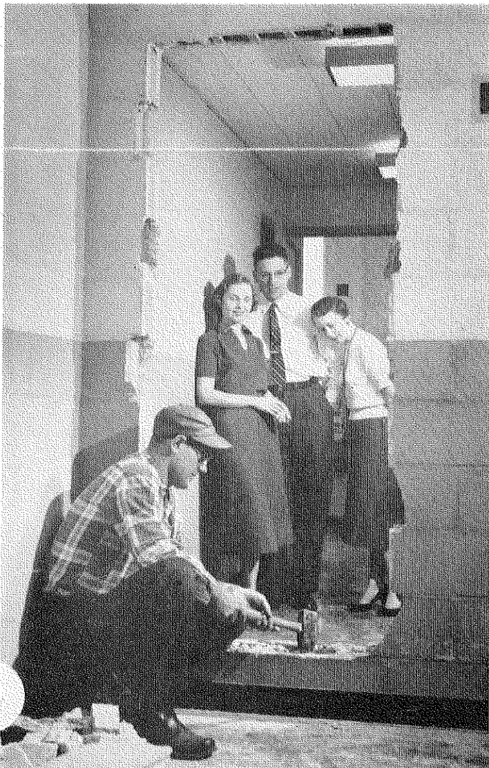
A NEW ENTRANCE into the technical library in the X-710 Building has been established for the convenience of individuals assigned to other parts of the building. Here G. L. Neal, utilities maintenance department, is removing the last of cinder blocks preparatory to setting in the door frame. Watching in the background are, left to right, Beverly Schumacher, C. E. Kip, and Alice Pitts, of the technical library staff. The new doorway will allow personnel assigned to the second floor of the X-710 Building to go into the library without first having to go down stairs, crossing the lobby, and climbing the stairs leading to the library.
