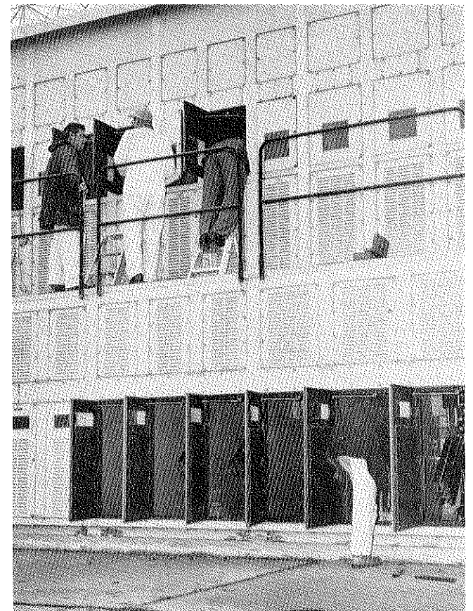
THE PROBLEM!! Loss of production resulting from the breakage or failure of any of the 756 wooden operating rods located in X-533 Electrical Switchyards. THE SOLUTION!! Replace them with a plastic (resin) rod which has greater mechanical and electrical qualities.
