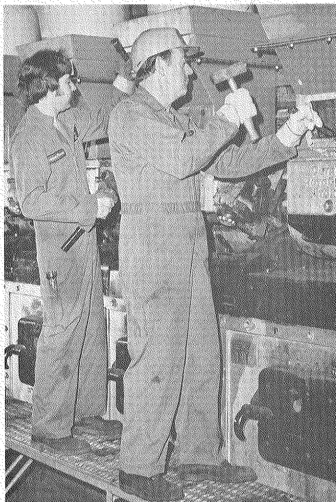
Ray Large and Cliff Thomas, pictured above left to right, fight a constant battle to keep the frozen coal moving through the stokers. During the winter, 12 of the stokers pictured above are in constant operation.
