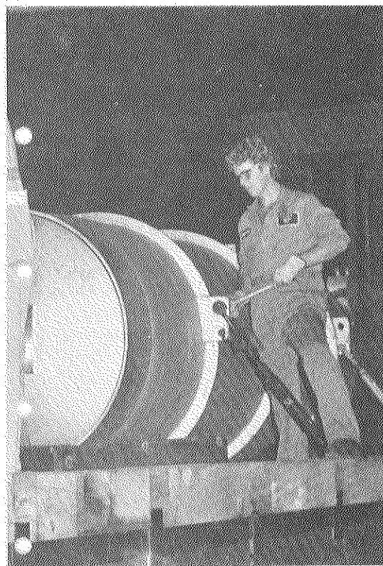
Instant awareness of proper safety and quality control by Richard Bussa make sure that all tie downs are checked before the railcars holding the cylinders
